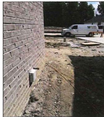
Clear pathway from meter location to gas main.
