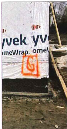
Meter location marked with a G.
