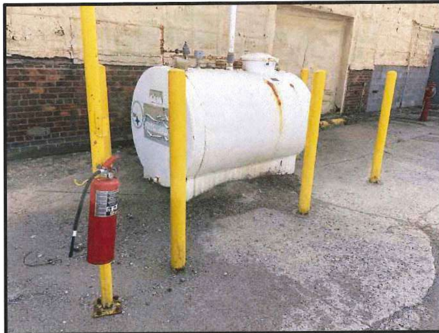
PARCEL A, ABOVEGROUND DIESEL STORAGE TANK (~500-GALLON) OBSERVED NEAR WESTERN EXTERIOR OF SUBJECT BUILDING 1
