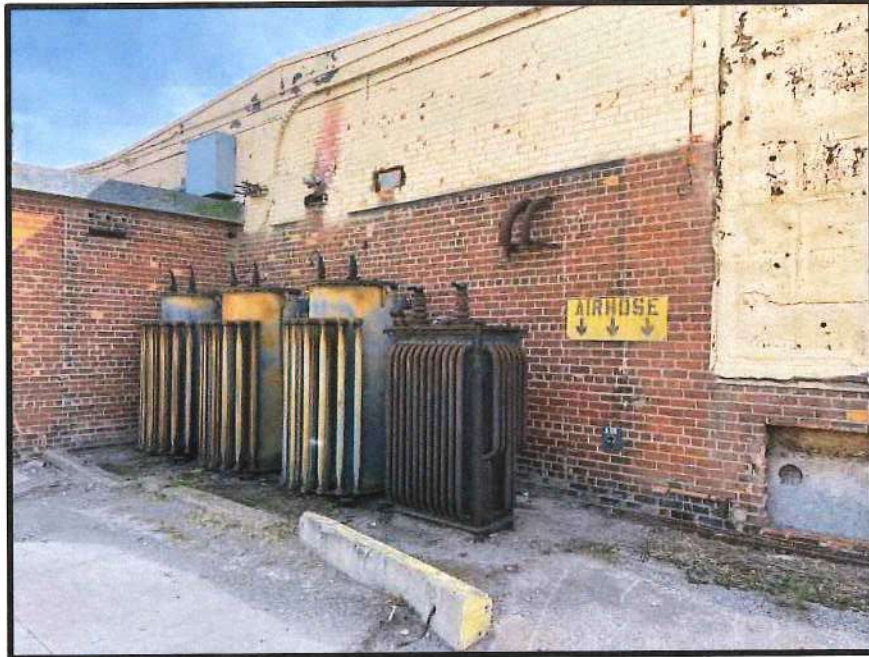
PARCEL A, VIEW OF TRANSFORMERS WITH STAINING NEAR WESTERN EXTERIOR OF SUBJECT BUILDING 1
