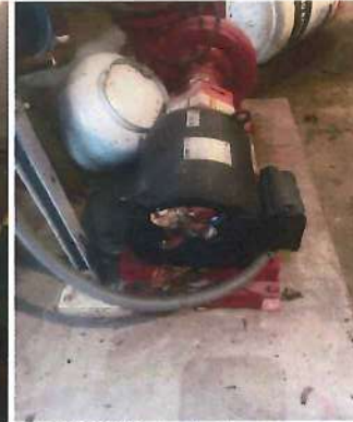
Pic#5 HWT circulating pumps debris pulled into propeller
