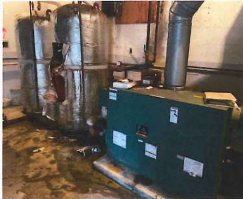
Pic #4: storage tanks and domestic HWT boiler
