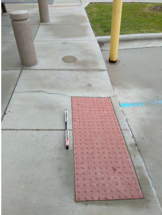
Running and Cross Slopes Checked
