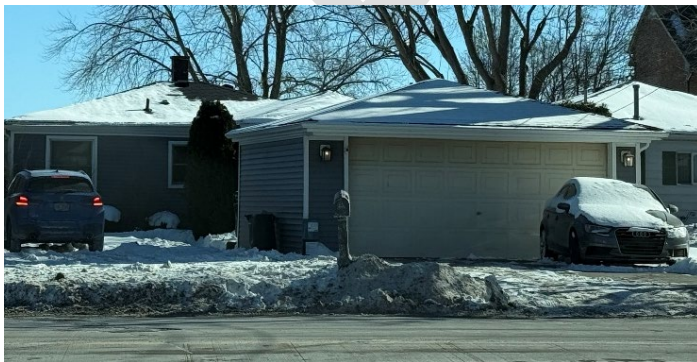
Figure 1 - Snout homes – Not permitted
