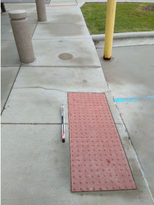
Running and Cross Slopes Checked
