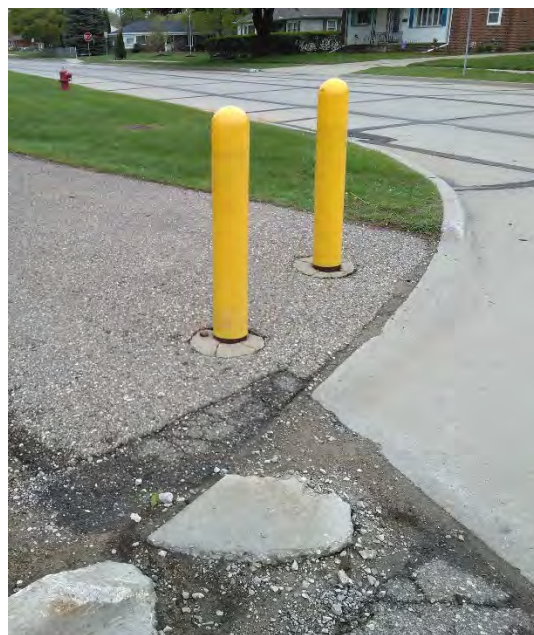
Clearances Checked at Pathways
